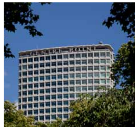
Centrepoint in London has recently been acquired by new owners who need to find a way of getting an income from empty office floors. One option would be conversion to residential.
