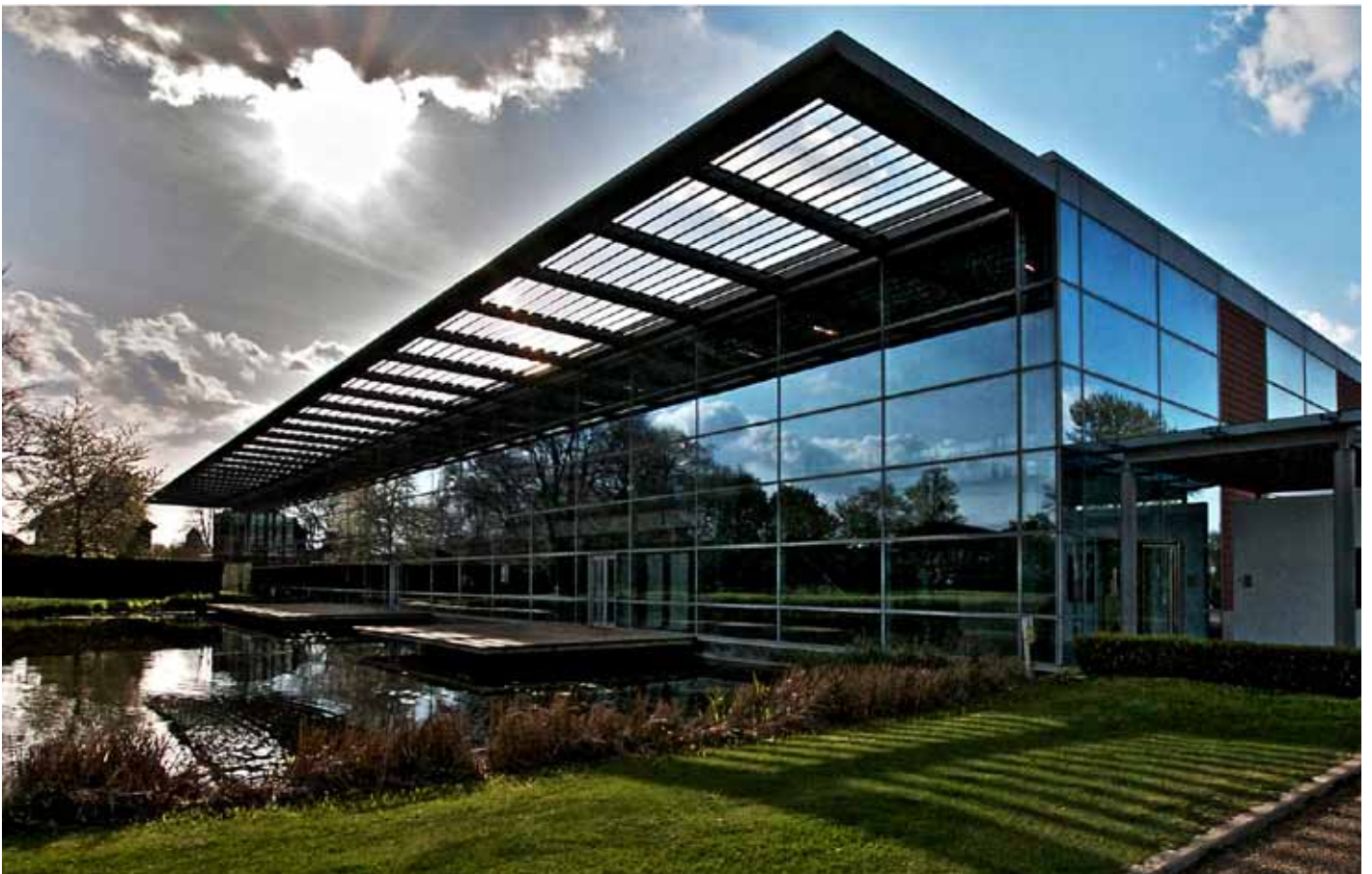
The da Vinci Building, Melbourn Science Park, Cambridge. GVA is providing leasing advice on this 41,000 sq ft office headquarters scheme.
